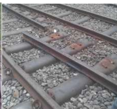
PLATE F: Accident encountered at Iddo rail track Lagos
